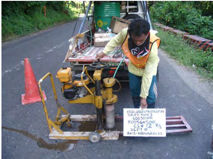
Southern Samar Coastal Road Project (Package III) Southern Samar Region
